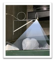
All the system components are designed not only to dispense the enzyme in a timely and precise manner, but also to ensure that the chemical covers the entire dumpster area by using a full cone pattern sprayer at the appropriate angle and height. The spraying components are attached to a 24-inch-long bracket to reach the center of the dumpster.
